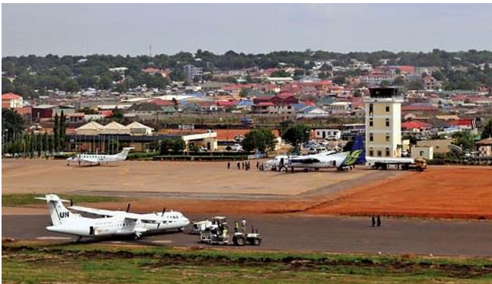
Figure 78. The Juba international airport.
