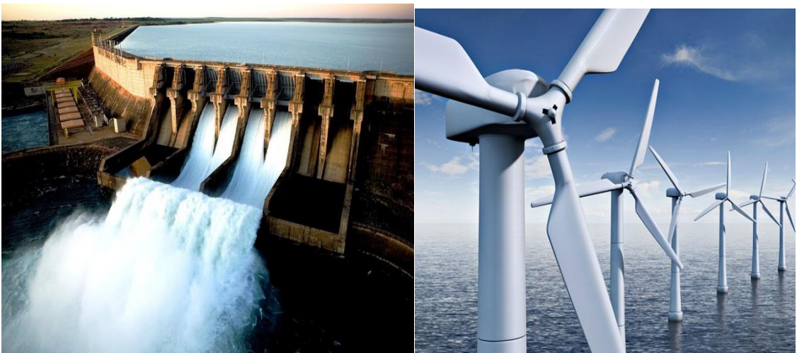
Figure 125. A hydroelectric dam and a wind farm.
