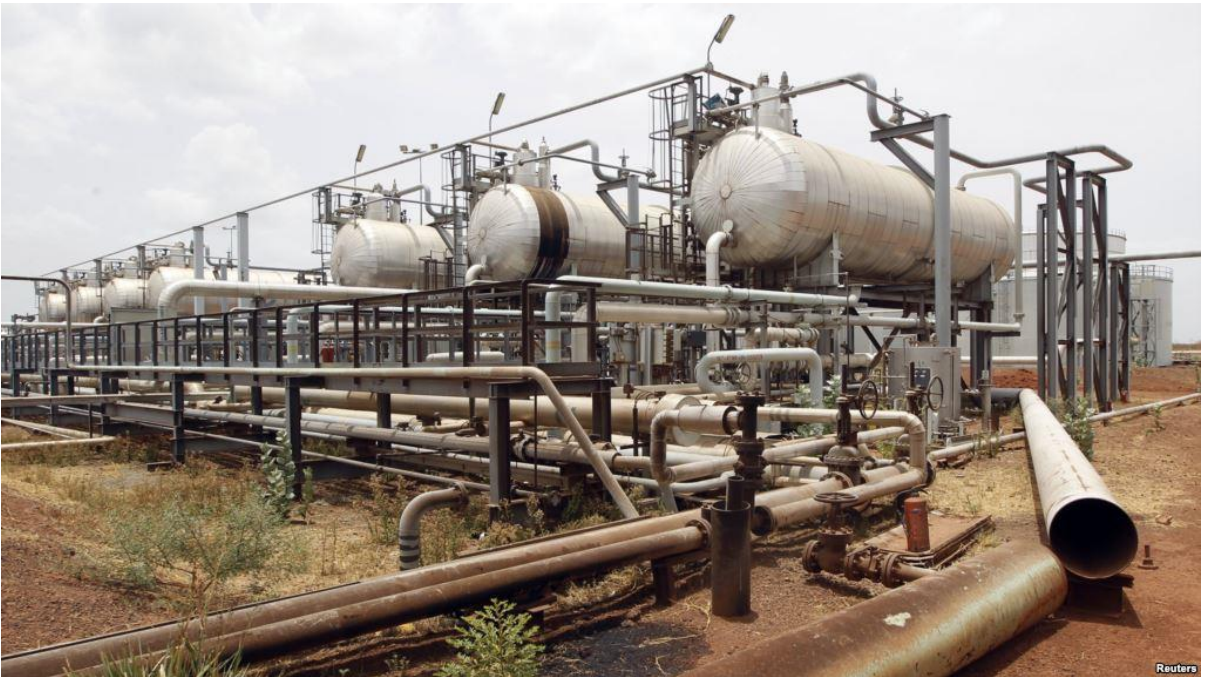
Figure 67. An oil facility in Unity state, South Sudan
